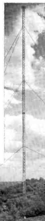
Slender 275-foot insulated tower for AM radio
